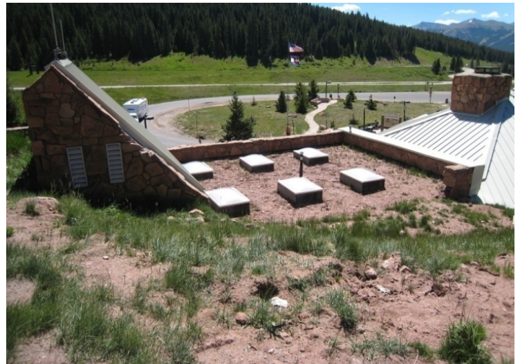
The Vail Pass Rest Area was built into a hill to help insulate the building, reducing heating and cooling costs. (Courtesy of CDOT)
