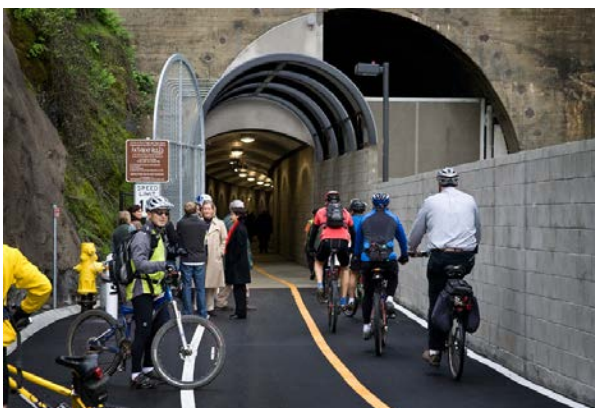
The Cal Park Hill Tunnel in Marin County connects a multi-use path to the Larkspur Ferry Terminal via a reconstructed railroad tunnel. (Courtesy of WalkBikeMarin)
