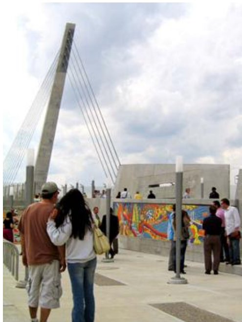
A pedestrian bridge reconnects Mexicantown and integrates community art into the project. (Courtesy of FHWA)
