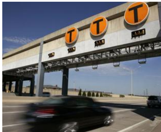
Analysts determined that implementing a toll system on existing freeways would not have disproportionately high and adverse effects on nearby EJ populations. (Courtesy of FHWA)
