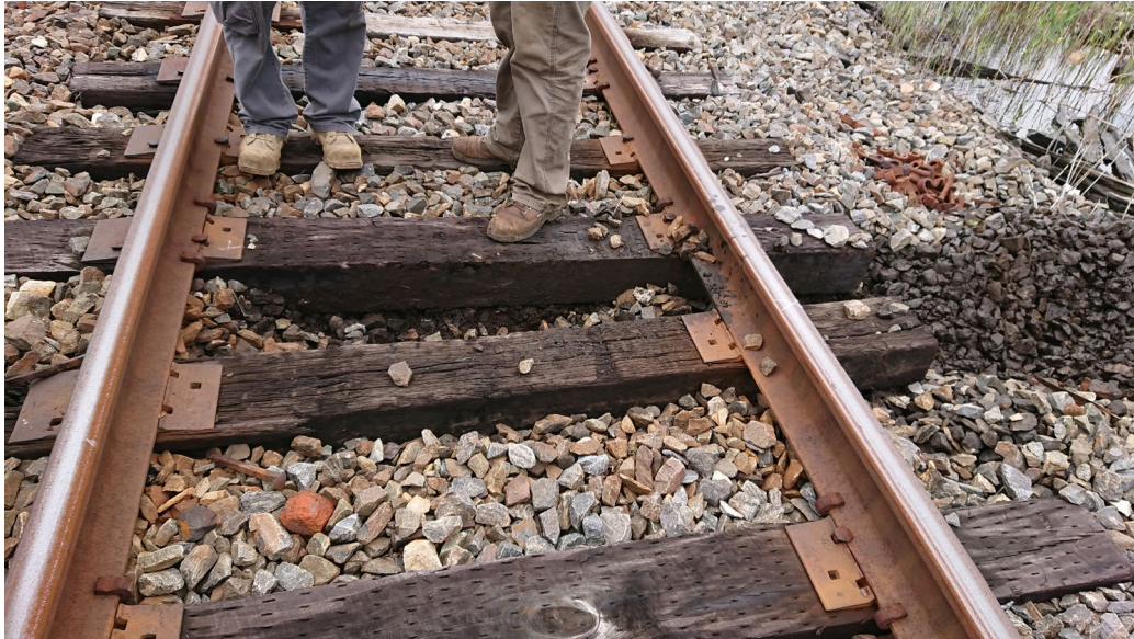
Figure 21 – Deliberate Ballast-in-Crib Height Change
