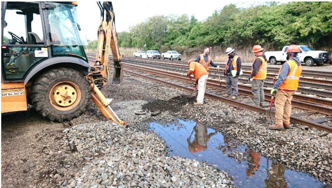
Figure 10 – Deliberate Changes to Ballast Level
