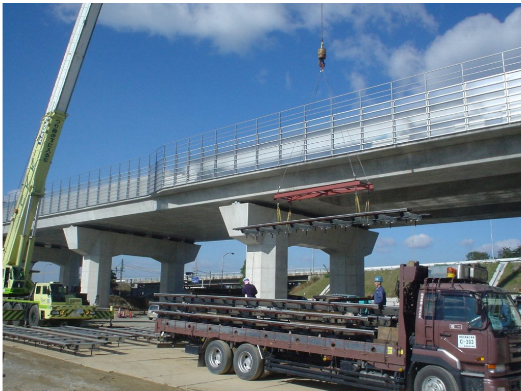
Figure 48: Guideway Sections Ready for Transport on the Guideway
