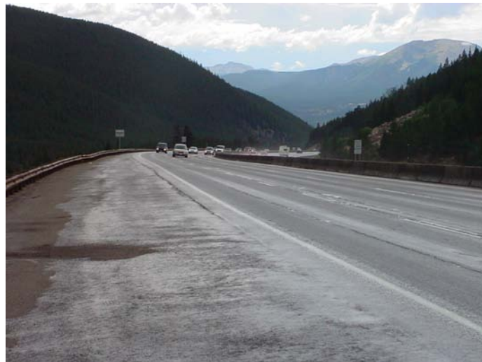
Figure 21: I-70 Westbound west of Eisenhower-Johnson Memorial Tunnel
