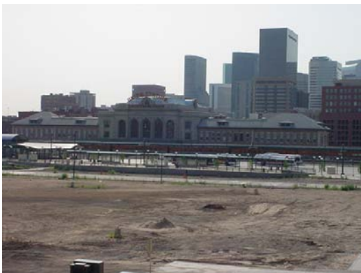
Figure 3: Denver Union Terminal
