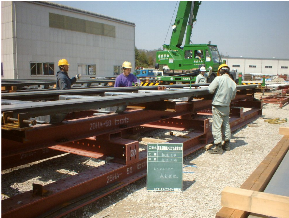
Figure 46: Levitation Rail Section Assembly Prior to Installation
