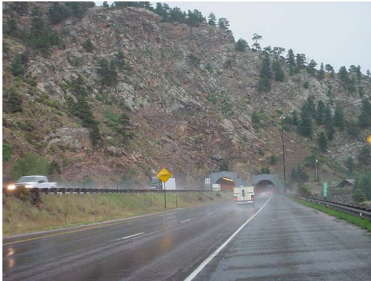
Figure 17: I-70 Eastbound at Twin Tunnels
