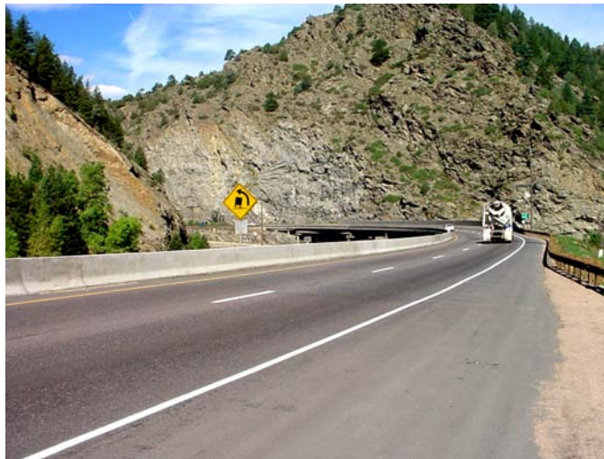
Figure 16: I-70 Westbound at base of Floyd Hill
