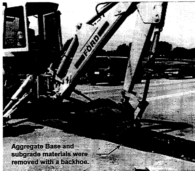
Figure 2.4 - Removal of Aggregate Base
