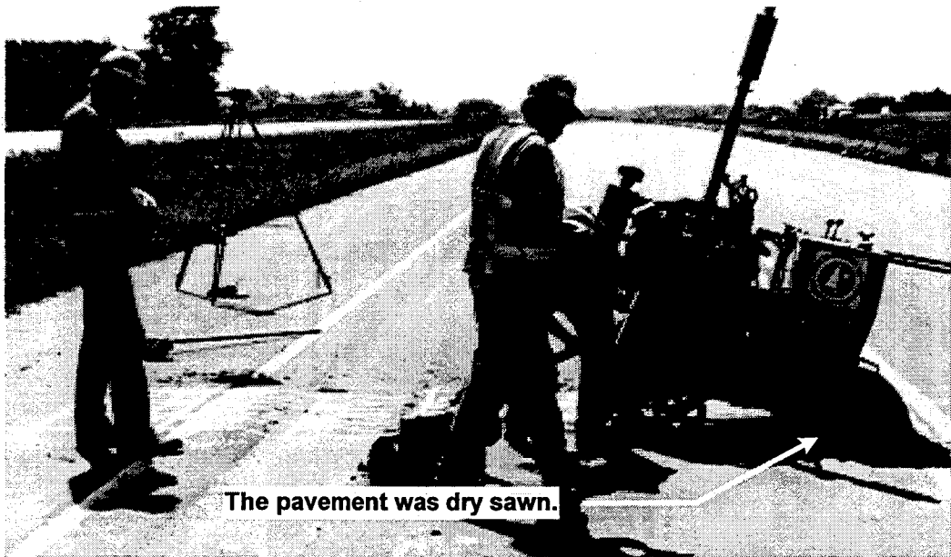
Figure 2.2 - Dry Sawing of Pavement
