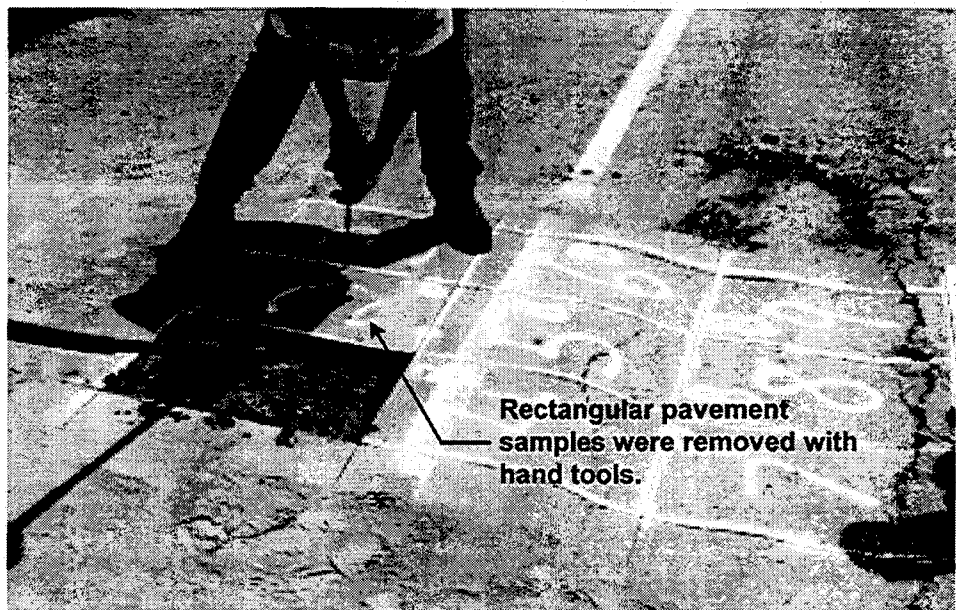
Figure 2.3 - Removal of Rectangular Pavement Sections
