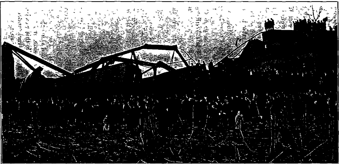
NO 2a—GENERAL VIEW OF WRECK, FIRST SPAN OF BRIDGE
