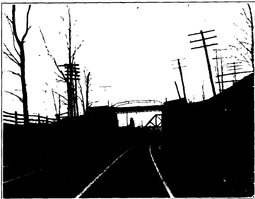
No. 5—View taken at a distance of two telegraph poles from highway bridge. flagman could not be seen from this point
