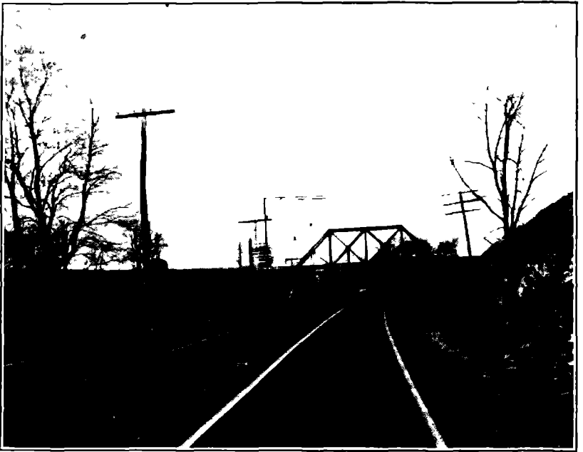
No 7 —View from a point under highway bridge, showing Trenton cut-off bridge and curve on which flagman was standing
