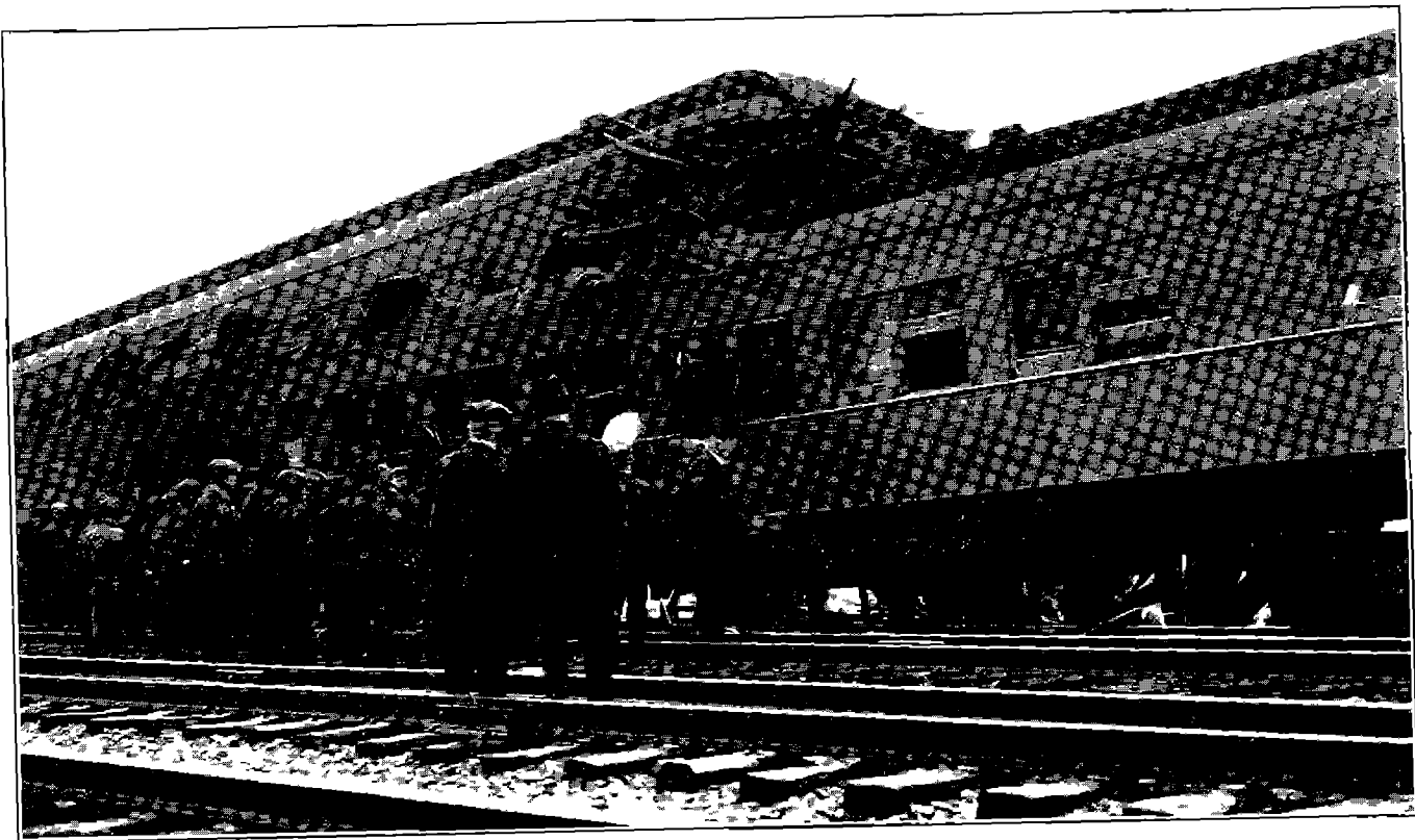
FIG NO 2—VIEW OF TELESCOPED CARS FROM NORTH SIDE OF TRACK
