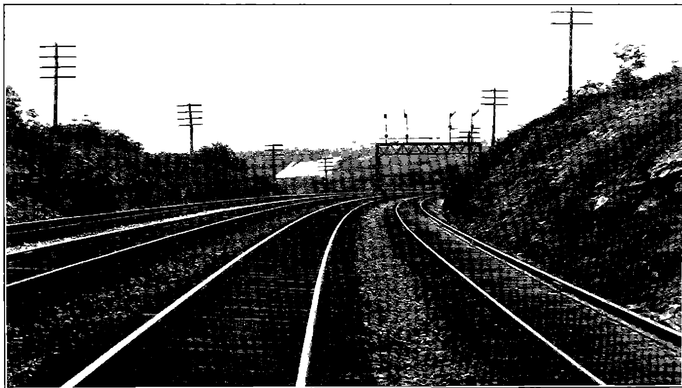
FIG. 1.—View of signal bridge 2012, taken on track 2 from point 16 rail lengths west of signal bridge
