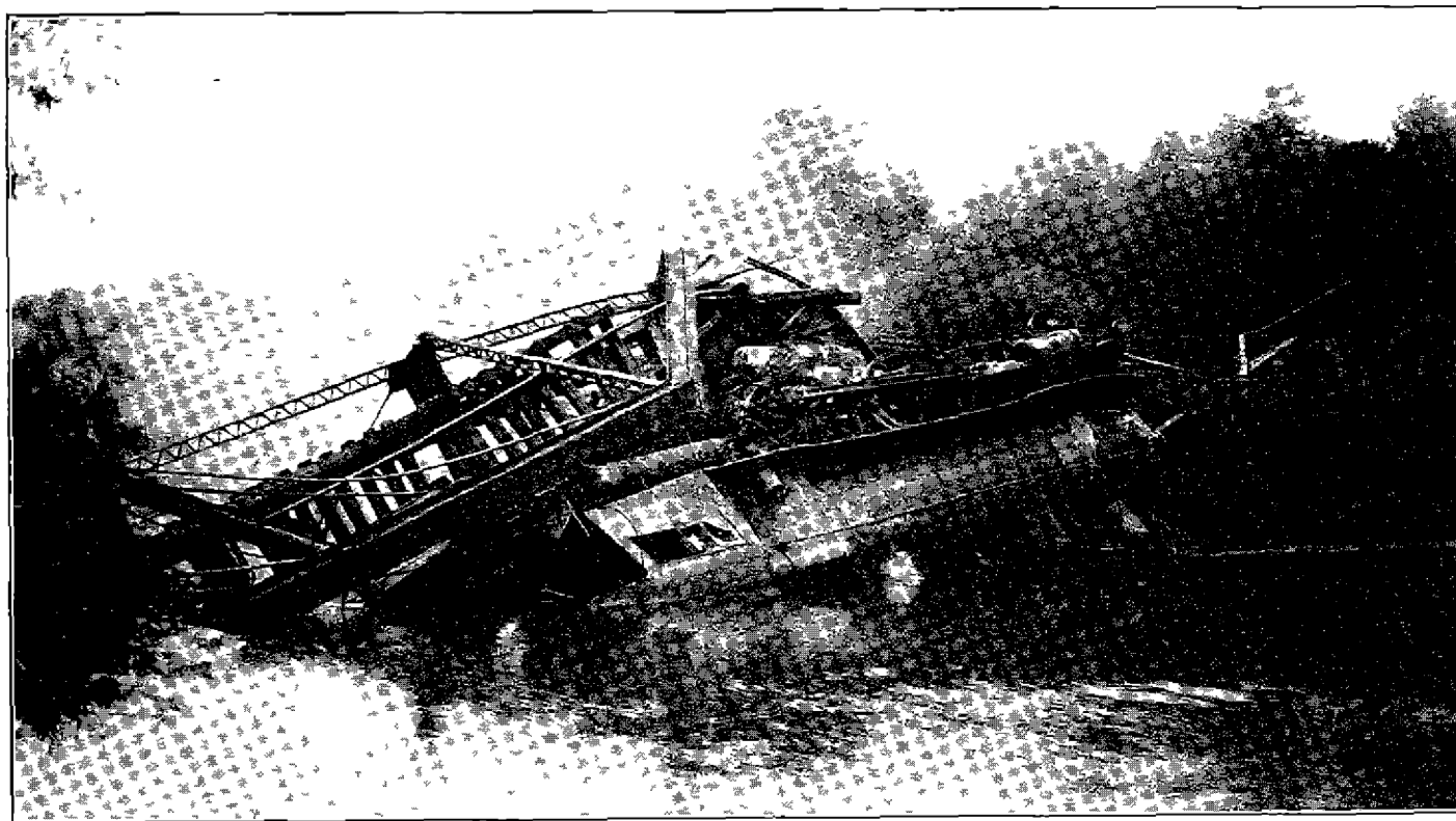
FIG 1—VIEW OF OVERTURNED ENGINE RESTING ON PARTIALLY DESTROYED CENTER PIER OF BRIDGE AND RIPRAP FOUNDATION SHOWING ALSO OVERTURNED TRUSSES OF BOTH SPANS FLOOR TIES NEARLY IN VERTICAL PLANE
