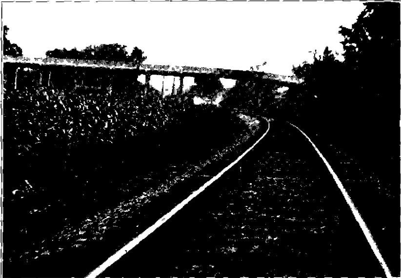
FIG. 5—VIEW OF TRACK AND OVERHEAD BRIDGE FROM DIRECTION TRAIN NO. 1 WAS TRAVELING
