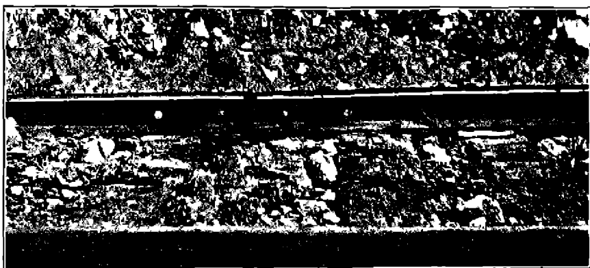
No 3 —Use of broken angle bar at joint
