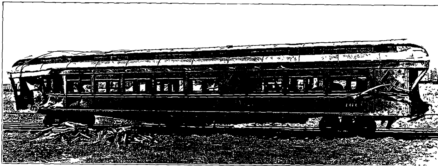
ILLUSTRATION NO 3 THE STEEL COACH AFTER REMOVAL FROM THE SCENE OF THE ACCIDENT SHOWING THE SIDE ON WHICH THE CAR RESTED AFTER THE COLLISION
