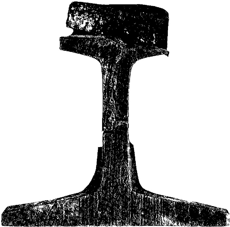
FIG 14—90 pound rail which failed near Friendship, N Y, Erie Railroad View of hot sawed end showing piped fracture in web, and horizontal shearing fracture in the head
