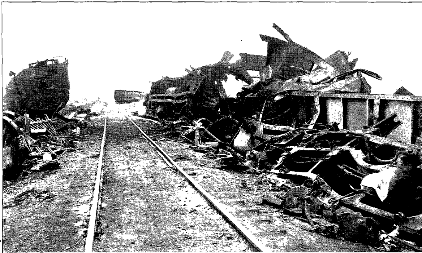
ILLUSTRATION NO 4—VIEW OF WRECKAGE AFTER TRACK WAS CLEARED
