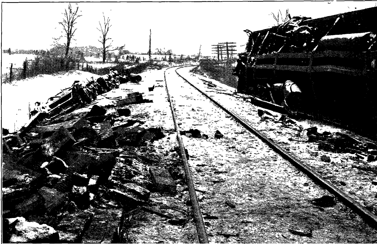
ILLUSTRATION NO 1—VIEW EASTWARD FROM POINT OF ACCIDENT
