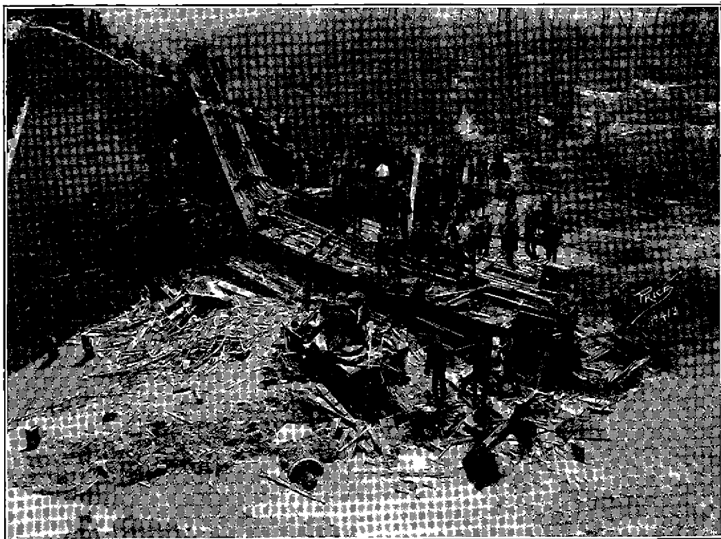
FIG 1—General view of derailed coach lying bottom side up on bed of Camp Creek with forward end leaning against east abutment of bridge
