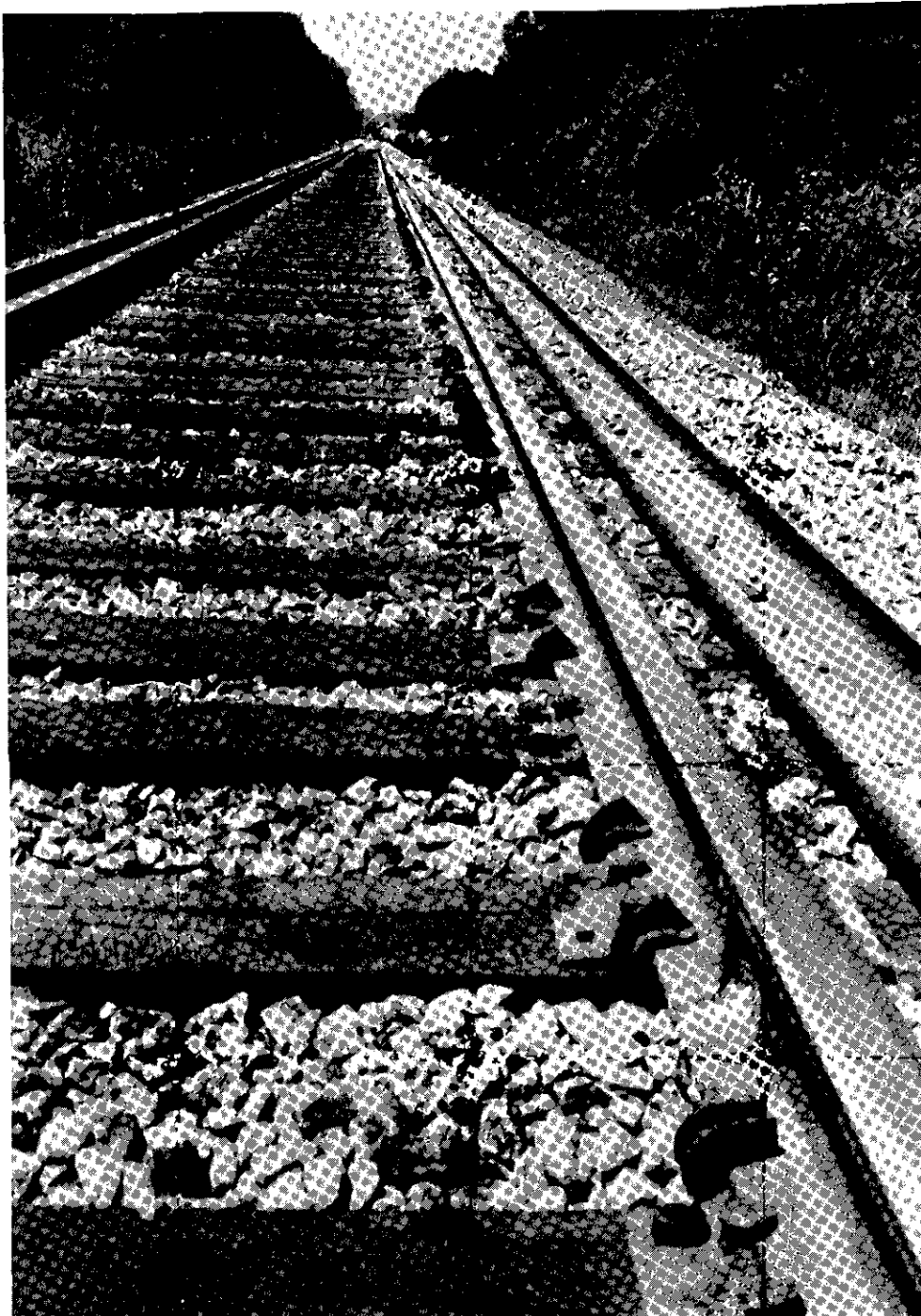
Figure 8.--The main track viewed facing south toward the derailment site at milepost 271.8 showing the field weld marking the location where the west rail was cut on May 7, 1985. Every second tie has been box anchored. New 136-pound rail to replace the existing 112-pound CWR is laying on the tie ends ready to be installed.
