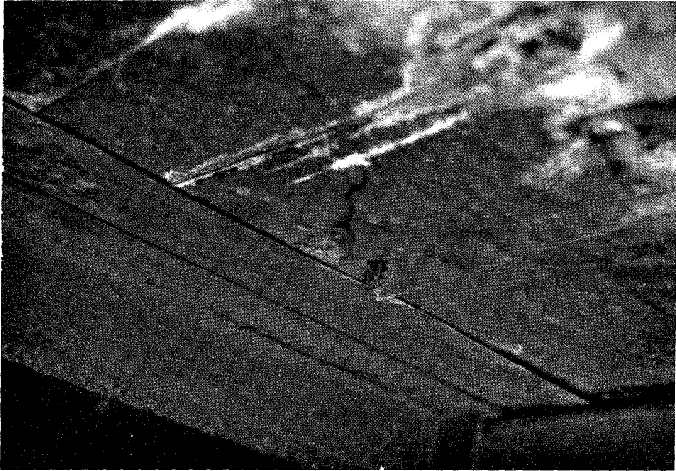
Figure 4. Broken floorboard of MKT 5394.
