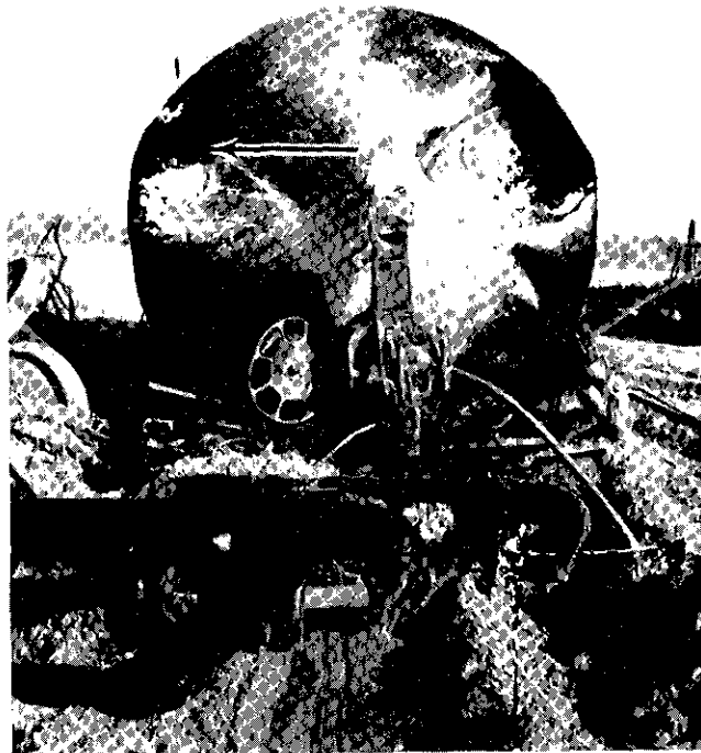
Figure 10.--Tank car ACFX 77725 in the Jackson accident. Note penetrated area of tank head shown at arrow.
