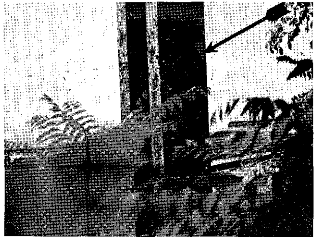
Figure 8.—Catenary Pole CP-F-137.12, 146 feet south of scene of accident.
