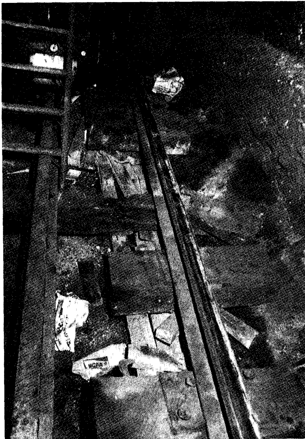
Figure 2.--Broken cross-tie and contractor's shoring, including wedges, at the derailment site.
