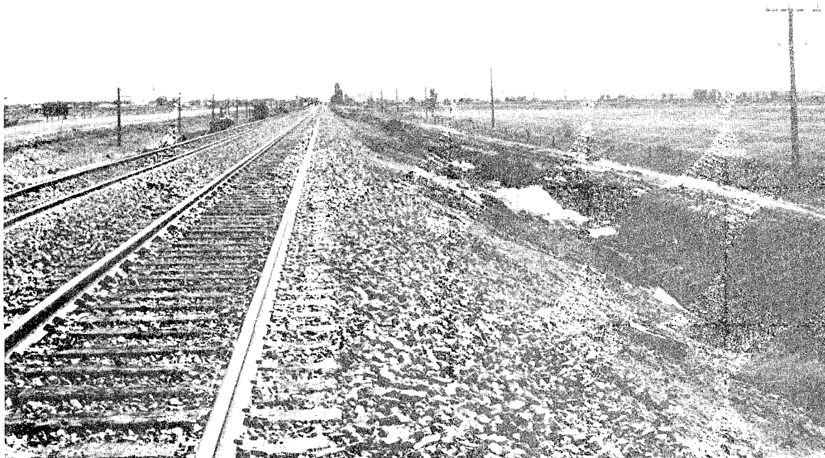
Figure 10.--Eastward view of accident site after track restoration
