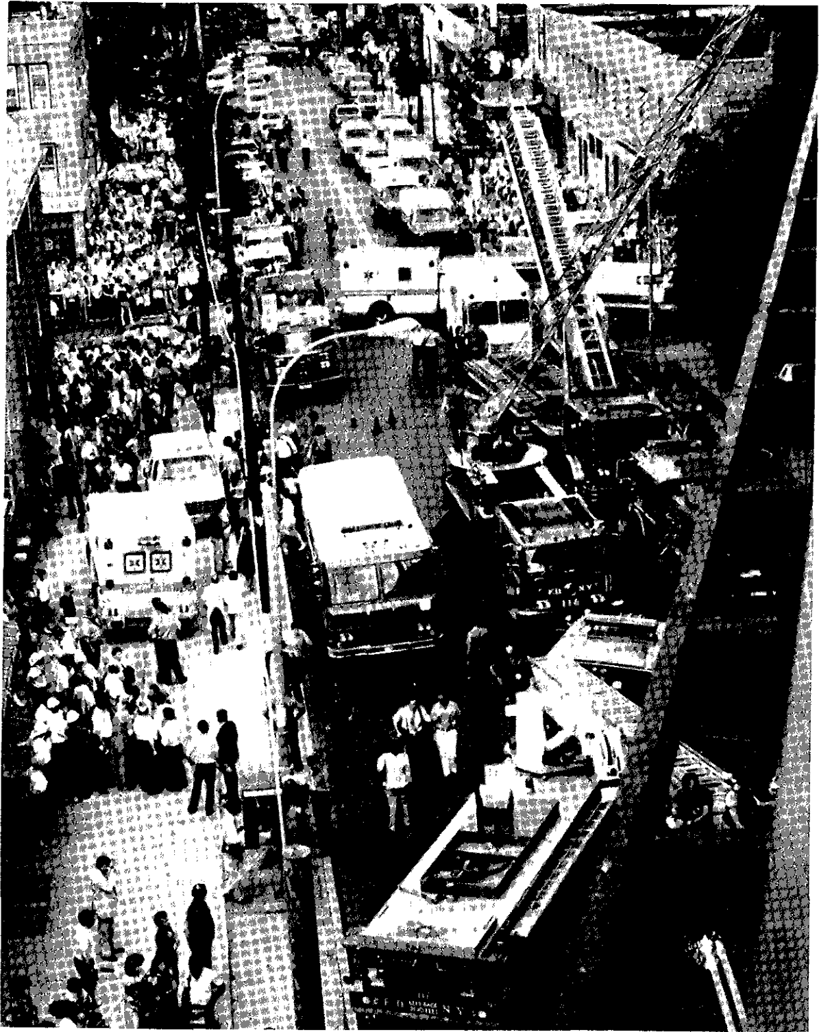
Figure 12.--Street scene below the viaduct at the accident site.
