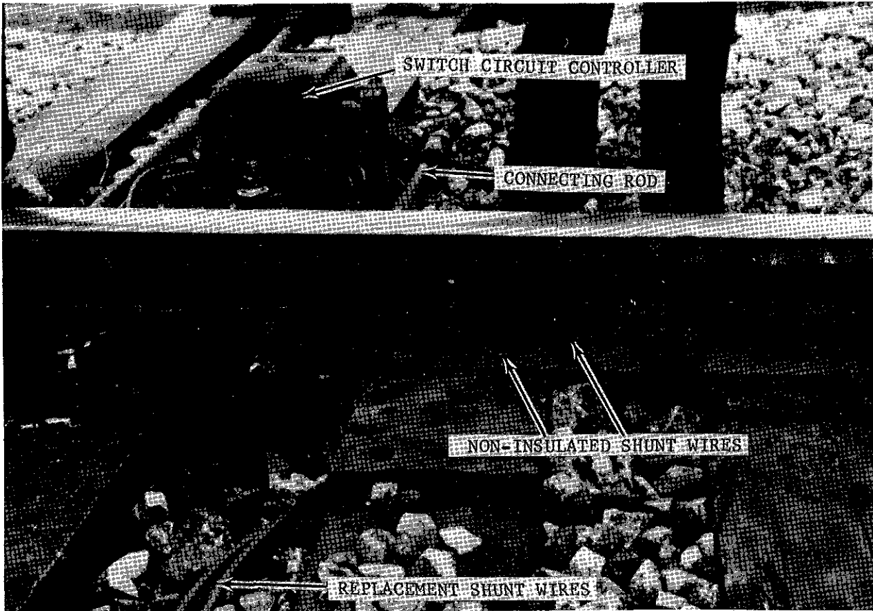
Figure 8.--Circuit controller and connecting rod. Note noninsulated shunt wires to be replaced.
