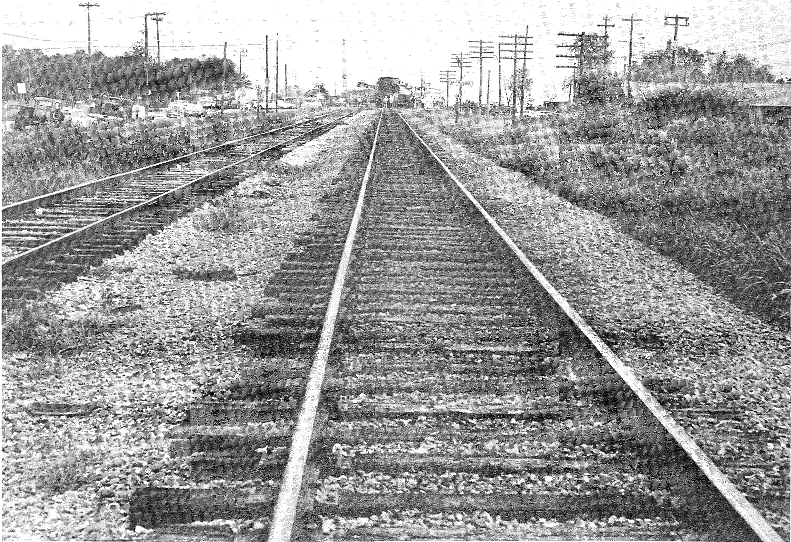
Figure 6 - View of tracks south of accident scene. The main track is on the right.
