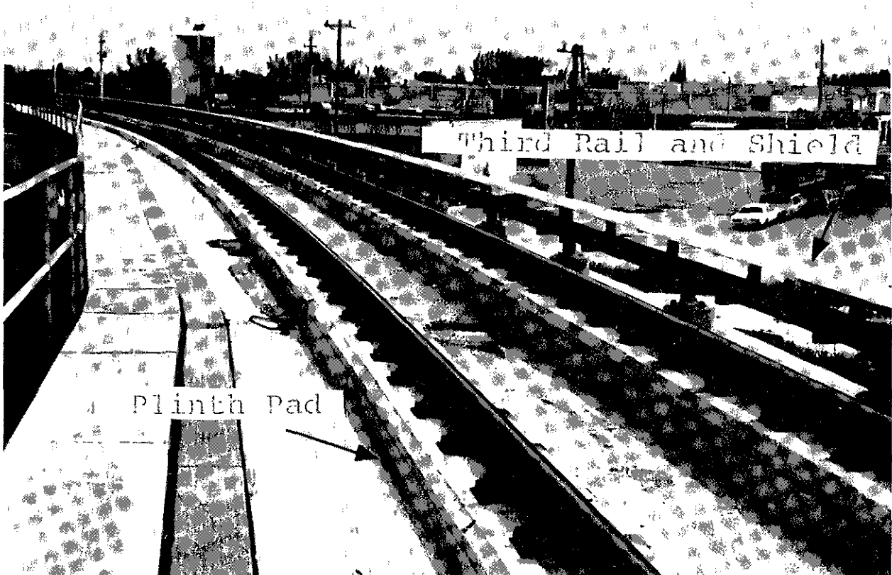
Figure 10.--Plinth pad on track.
