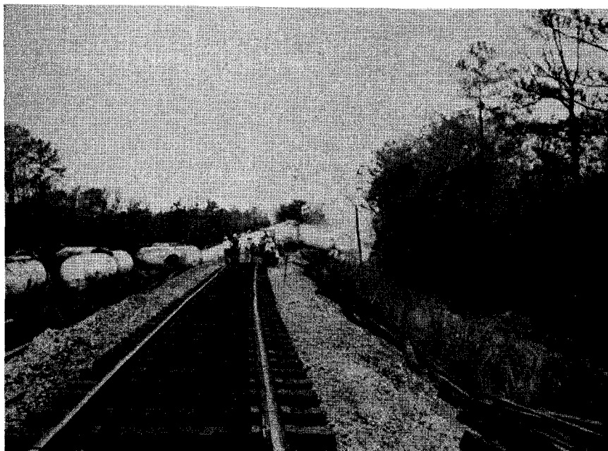
Track structure being restored.
