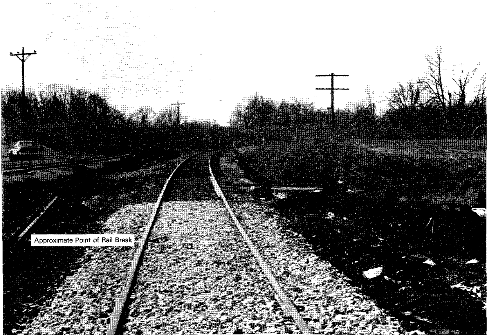
Figure 4.—View looking south from point of derailment.
