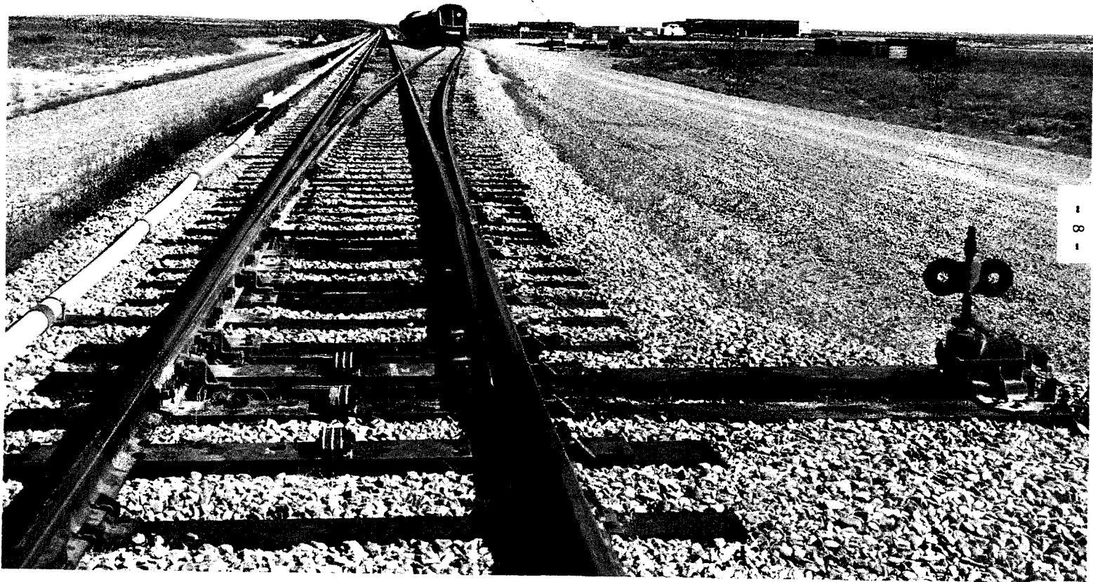
Figure 4. North access track switch, looking north. Switch is in "open" position. The SOAC's are visible at the collision point in the background.
