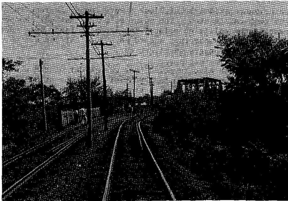
Figure 4. The operator of eastbound Block 4 had this view of the 6° curve approaching the point of collision on the arch bridge (center). There is a transit car 180 feet beyond the collision point, near the truss bridge (background), which is completely hidden by trackside vegetation.
