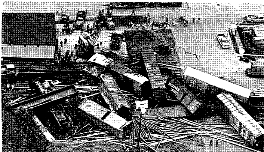
Extra 725 South approached from right. Locomotive of that train is under gondola car at left. Locomotive of Extra 675 South is under wreckage at center.
