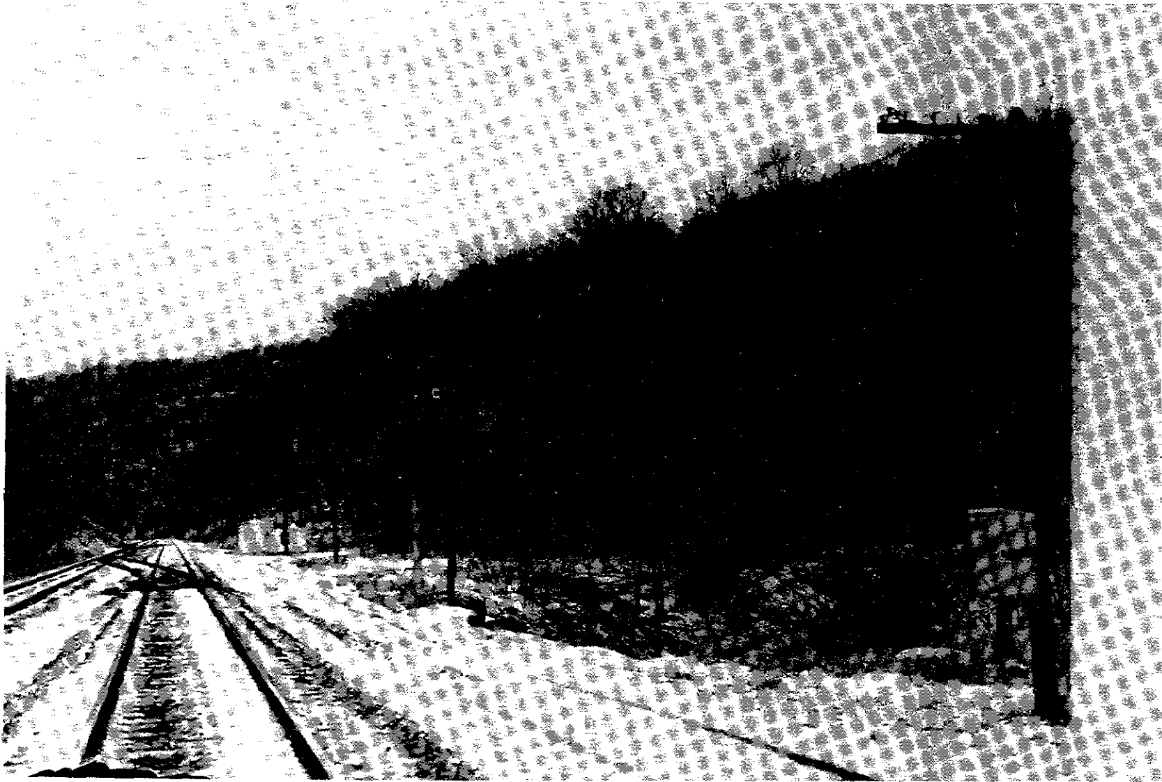
Figure 5.—Nonilluminated "C" light at CP Salts looking west. Signal lights are red indicating stop.
