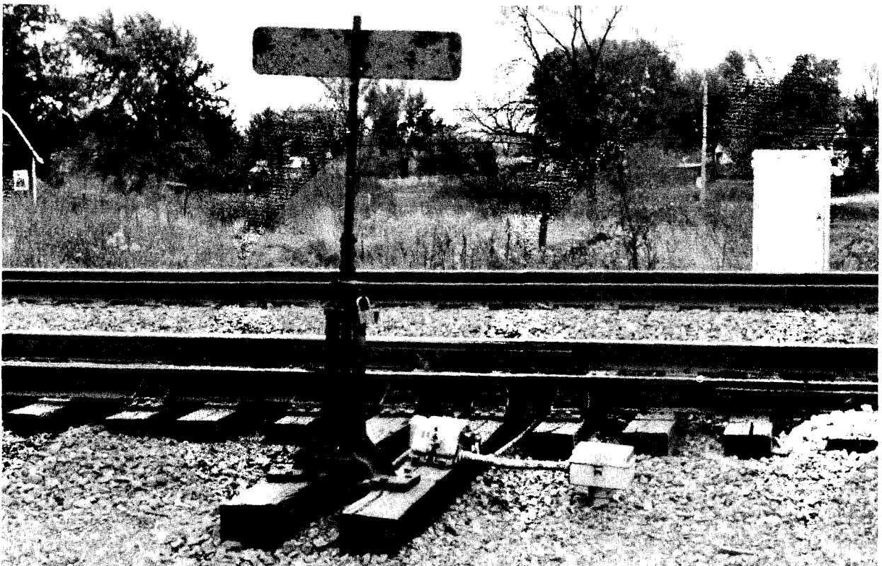
Figure 11.--West stub track switch banner.
