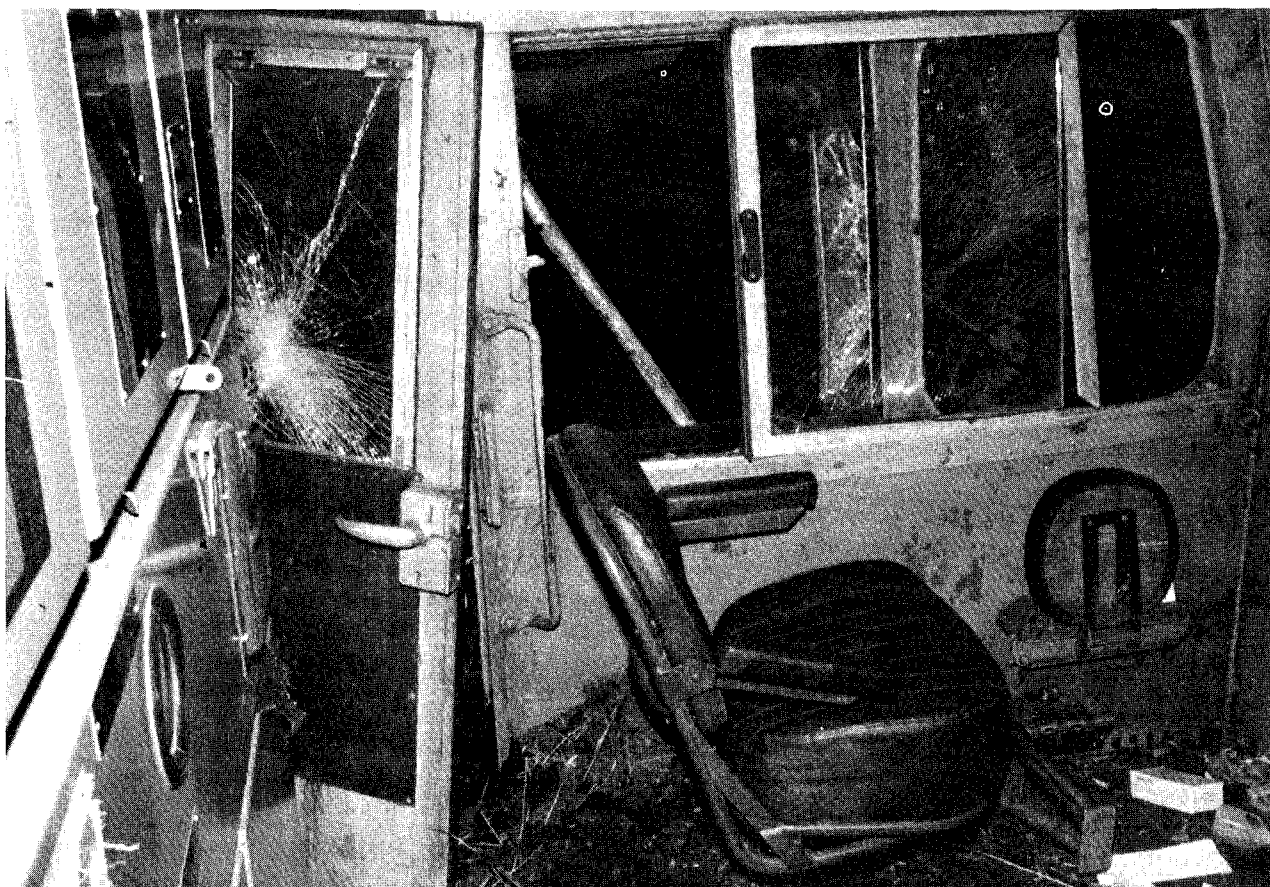
Figure 12 --Interior of the fireman's side of locomotive.
