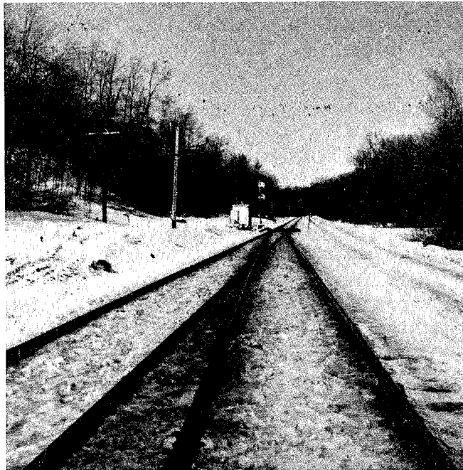
Figure 3. View of switch at Sherwin.
