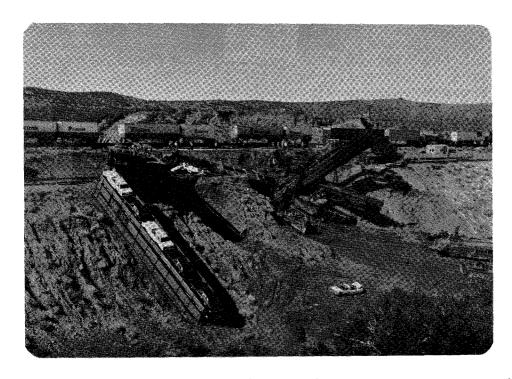
The momentum of the train carried the lead locomotive unit across the 95 foot washed out landfill and brought it to rest on the east edge of the area (as shown in the photograph). The three remaining locomotive units and the first six cars fell into the chasm created by the washout and immediately caught fire. The next ten cars were derailed and stopped on or near the track structure.
