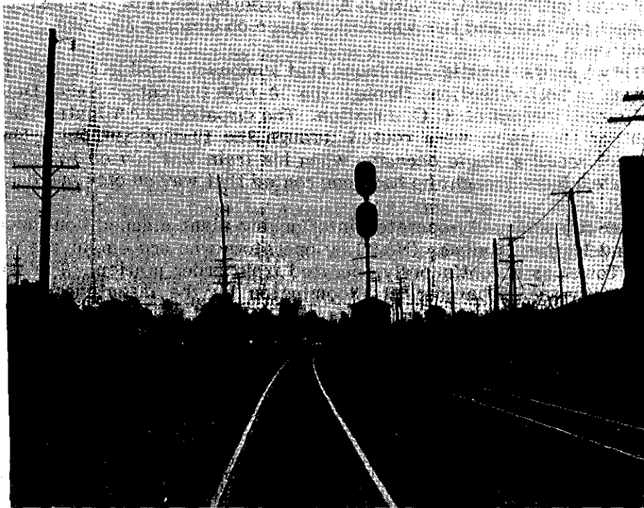
Figure 1.--View from southbound train approaching the home signal and tower at Iles. Iles Avenue crossing is beyond the tower.
