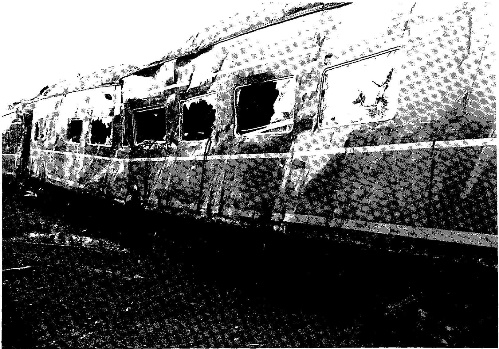
Figure 12.—Large observation type windows broken out when car 2616 overturned. Note outward distortion of broken glass in two nearest windows. The broken out windows became the floor of the passenger compartment as the car slid to a stop. At least one or as many as three passengers were ejected through these holes and were fatally injured.
