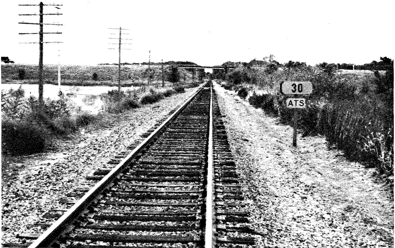
Figure 6.--New 30-mph speed-restriction and ATS signs installed in location of missing 30/25-mph speed-restriction sign on south side of track.
