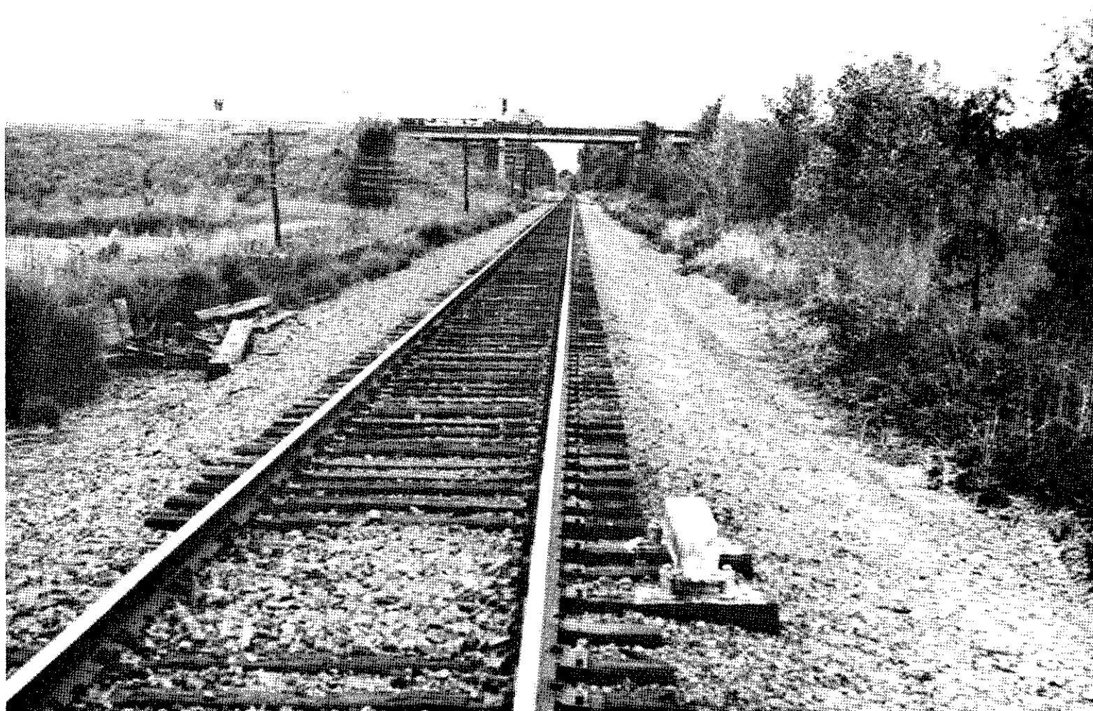
Figure 5.--Inert inductor to outside of right rail on south side of track.
