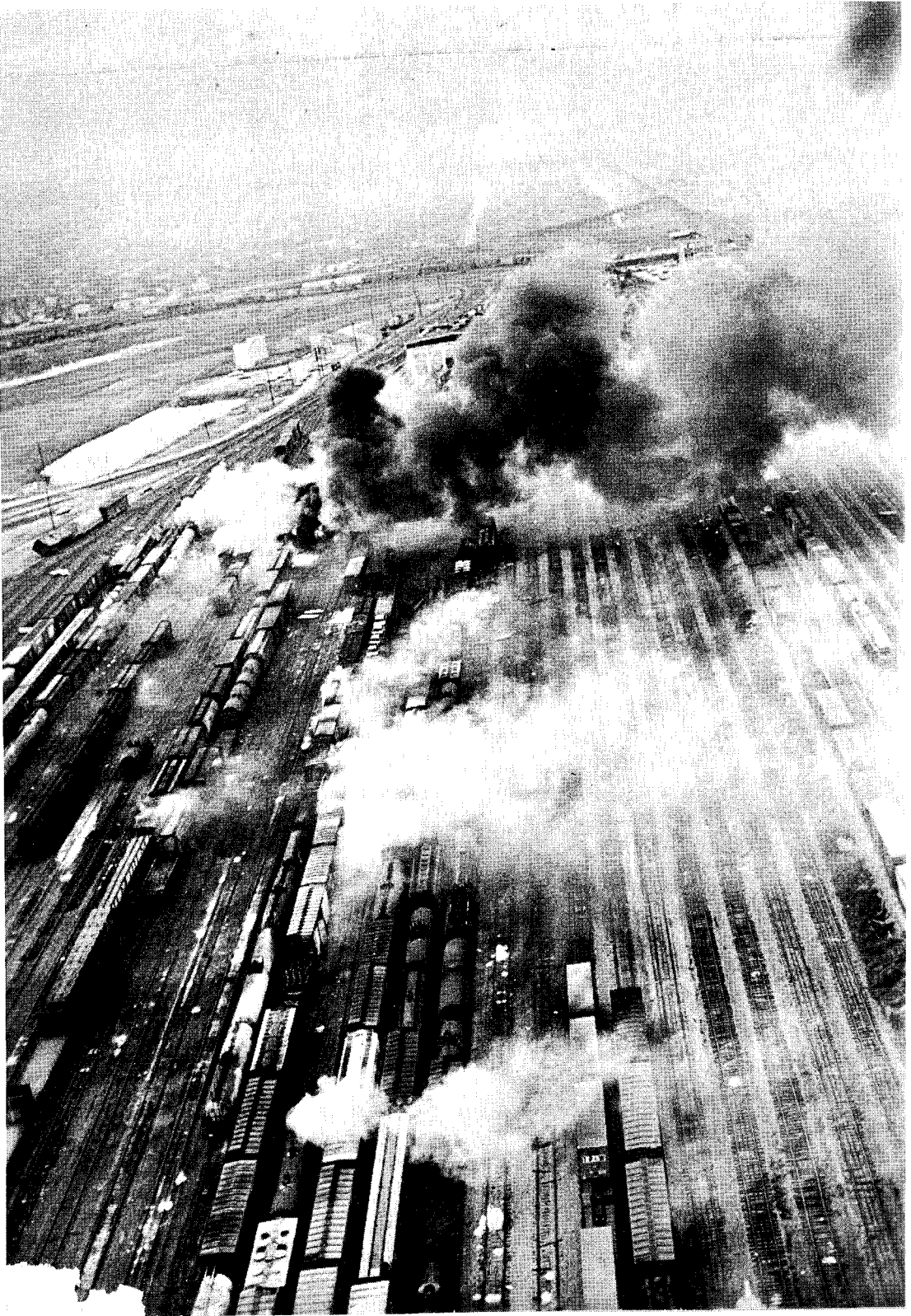
Figure 1. Alton & Southern Gateway Yard after the explosion.
