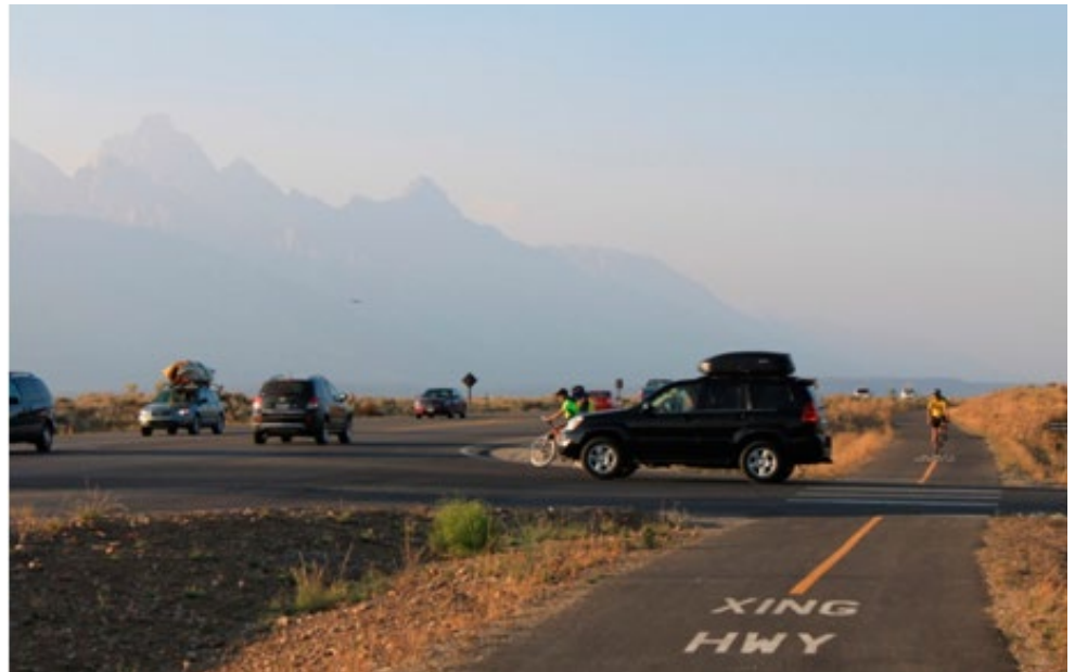
The crossing of a newly constructed shared use path near the intersection of Gros Ventre Road and Highway 89 in the Grand Teton National Park. IMAGE COURTESY of Elissa Goughnour, VHB.
