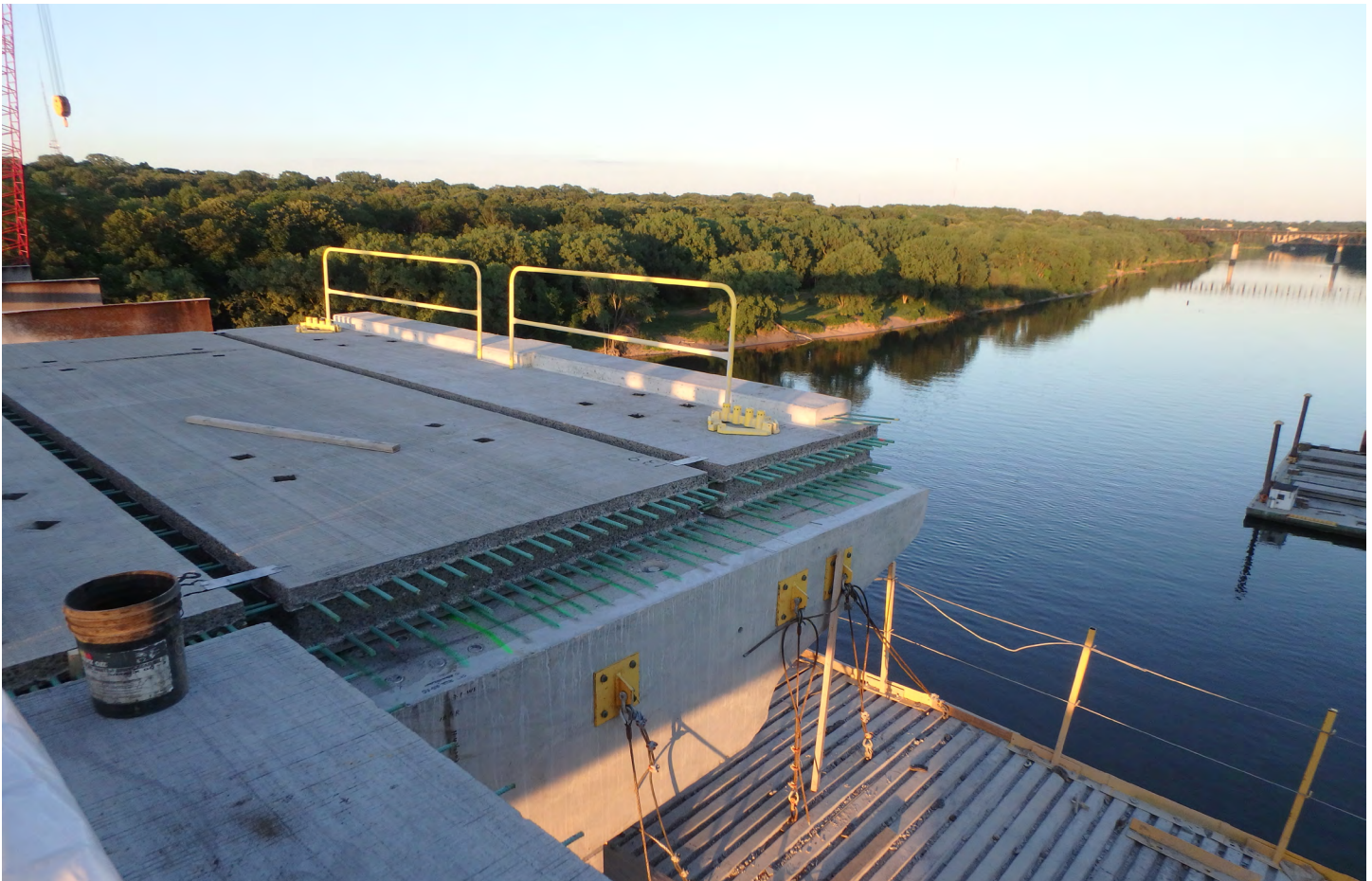
UHPC connection details make using prefabricated bridge elements simpler and more effective for accelerated bridge construction.
