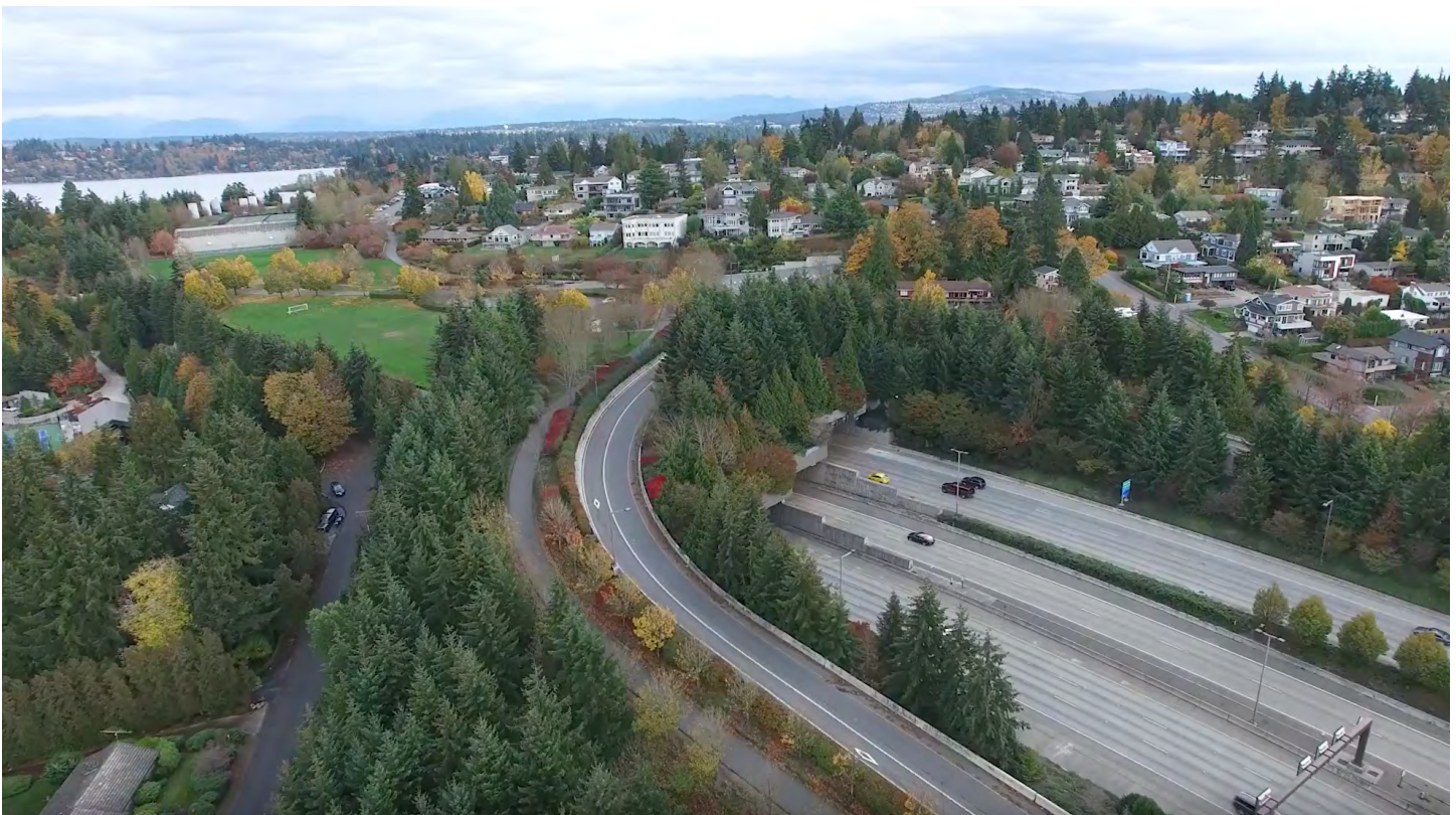
The lid over Interstate 90 on Mercer Island near Seattle, WA, enhances community connections with green space for a public park.
