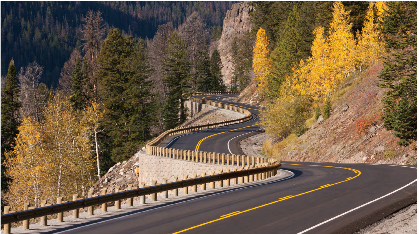
Employing a project delivery process that integrates environmental reviews and permitting can help achieve effective and efficient delivery of transportation projects.
