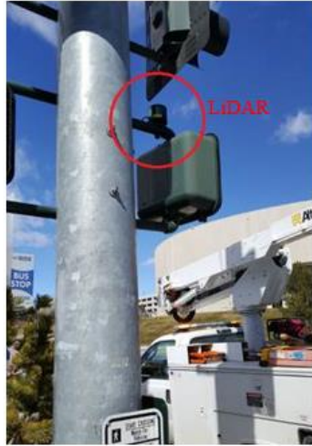
(a) Permanent installation (b) Temporary installation Figure 0-7 Different installation methods of roadside LiDAR sensors
