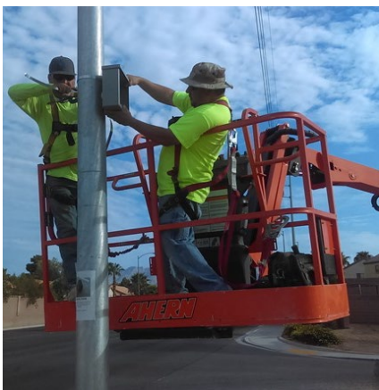
(a) Working on the communication box
