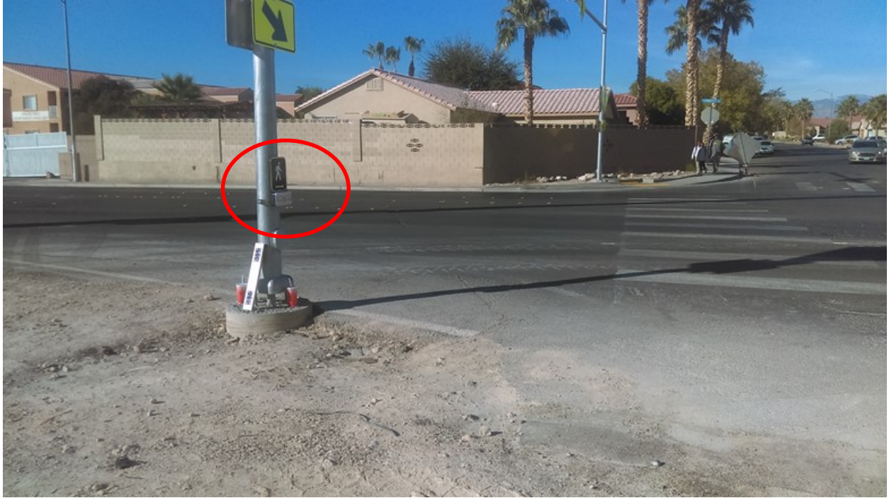
Figure 10 Infrared sensor for pedestrian detection
