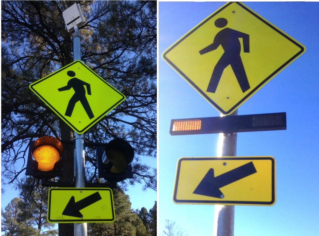
Figure 4 Circular and Rectangular Rapid Flashing Beacons
