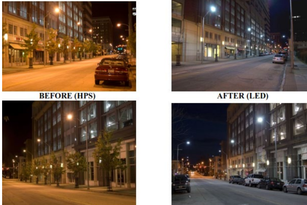
Figure 3 Before and after photos of the Street LED lighting
