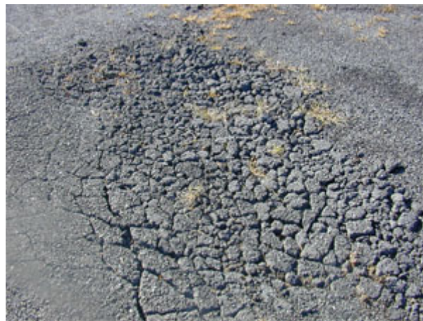
Figure 4 Alligator cracking in AC surface
