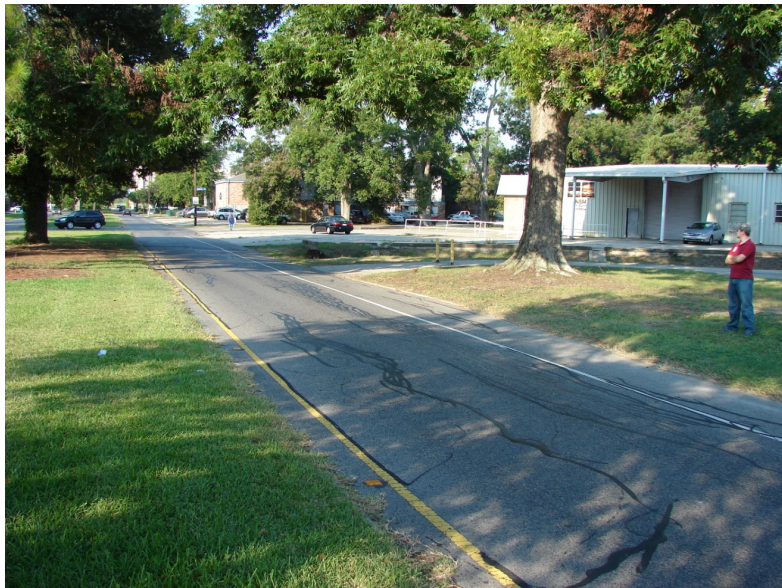
Figure 7 Multiple longitudinal cracks and subsidence: West Parker near LTRC
