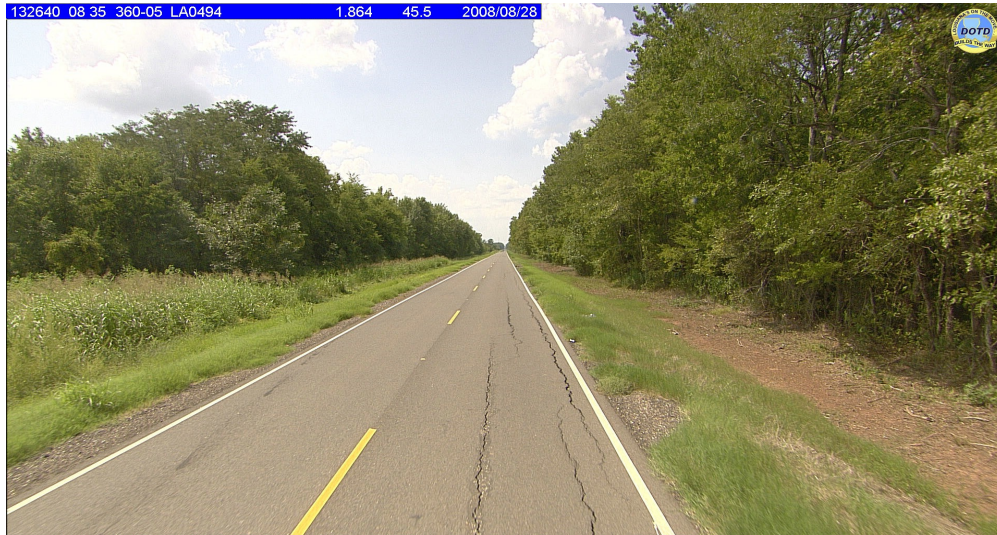
Figure 2 Multiple Longitudinal cracks: LA 494: CSLM 1.864
