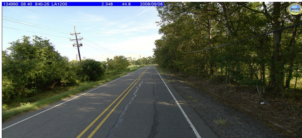
Figure 1 Longitudinal cracks: LA 1200: CSLM 2.348
