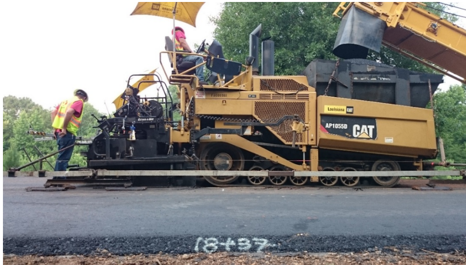
Figure 4 Paver stopped at 200-ft. calibration point
