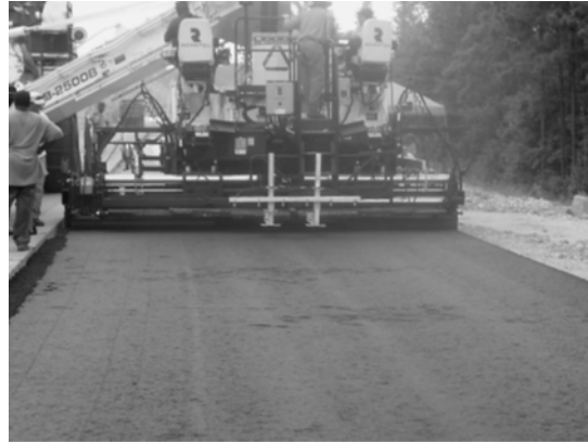
Figure 1 A prototype Pave-IR system on NCAT test track (Stroup-Gardiner 2004)
