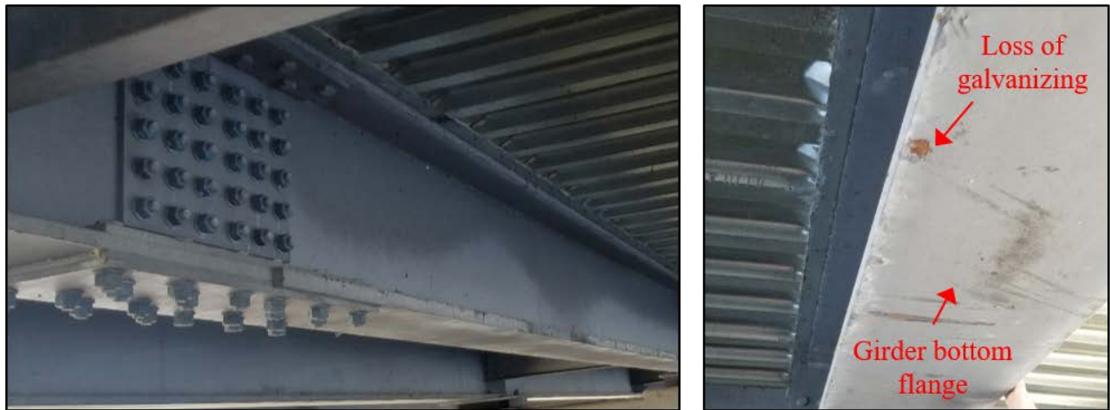
Figure 10. Visual Condition of Galvanized Weathering Steel Girder in March 2018: left, an example of the general condition; right, the only location exhibiting loss of galvanizing coating and showing the underlying weathering steel girder
