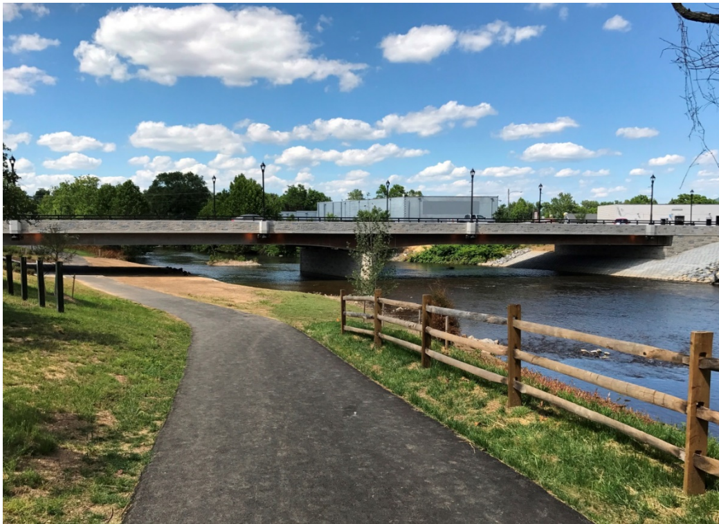
Figure 26. Route 340 Bridge With ASTM A709 Grade 50CR Steel Girders
