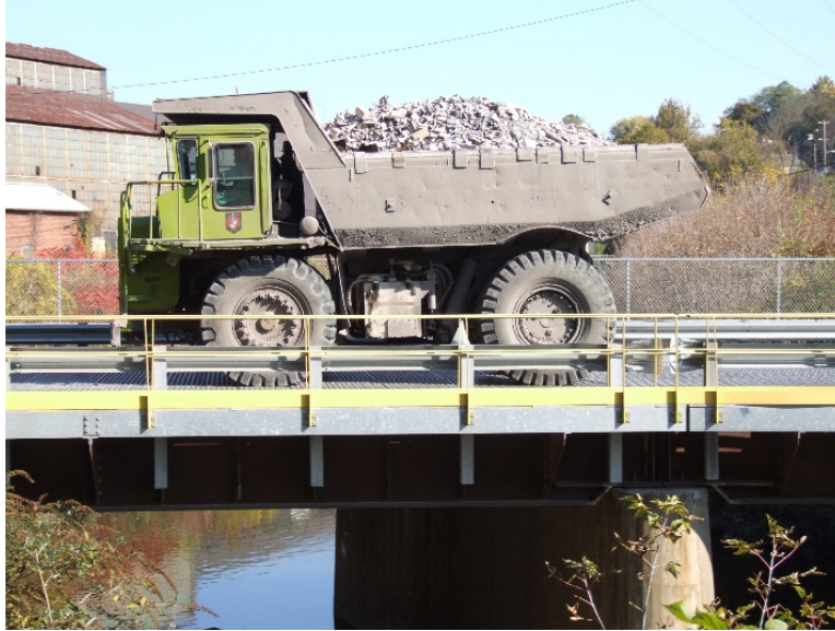
Figure 12. William G. Taylor Memorial Bridge Constructed Using ASTM A709 Grade 50CR Steel Plate Girders
