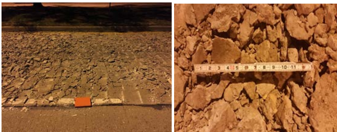
Figure 6. Particle Size After Rubblization (Before Rolling)
