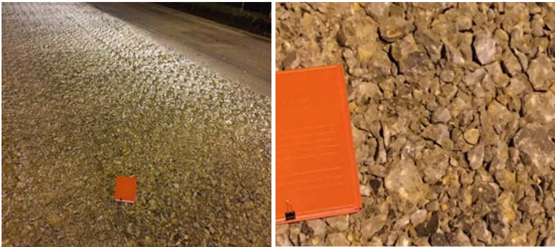
Figure 11. Final Rubblization Surface
