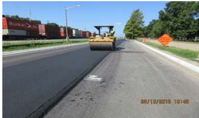
Figure 13. Placement of SM 12.5E Mixture
