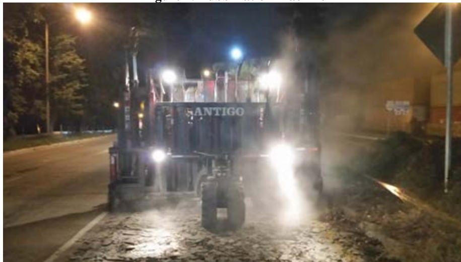
Figure 5. Rubblization Process
