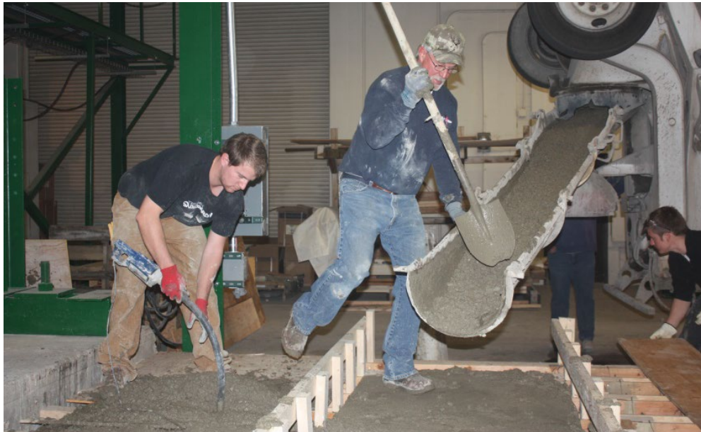
Figure 2.13 Concrete placement
