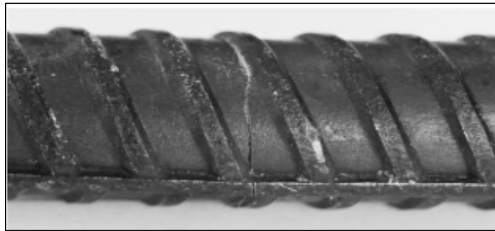
Figure 1.6 Fatigue crack in rebar with initiation at intersection of longitudinal and transverse ribs (Derkowski, 2006)
