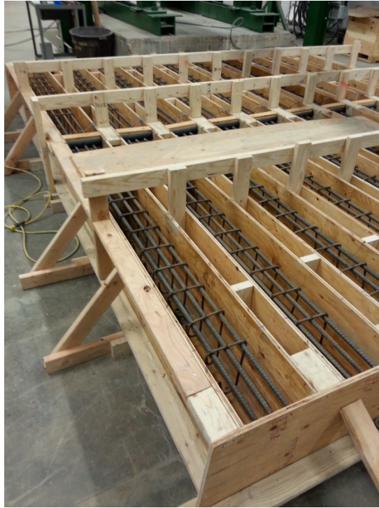
Figure 2.10 Braced plywood and lumber form-work
