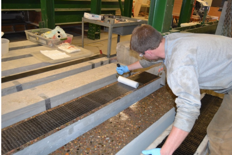
Figure 2.15 Hand-layup process of Tyfo SCH-41 CFRP sheets and beams 4 and 5
