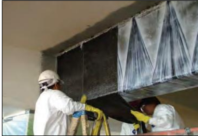
Figure 1.5 CFRP fabric sheet wet layup application to girder (CPS Construction Group, 2011)
