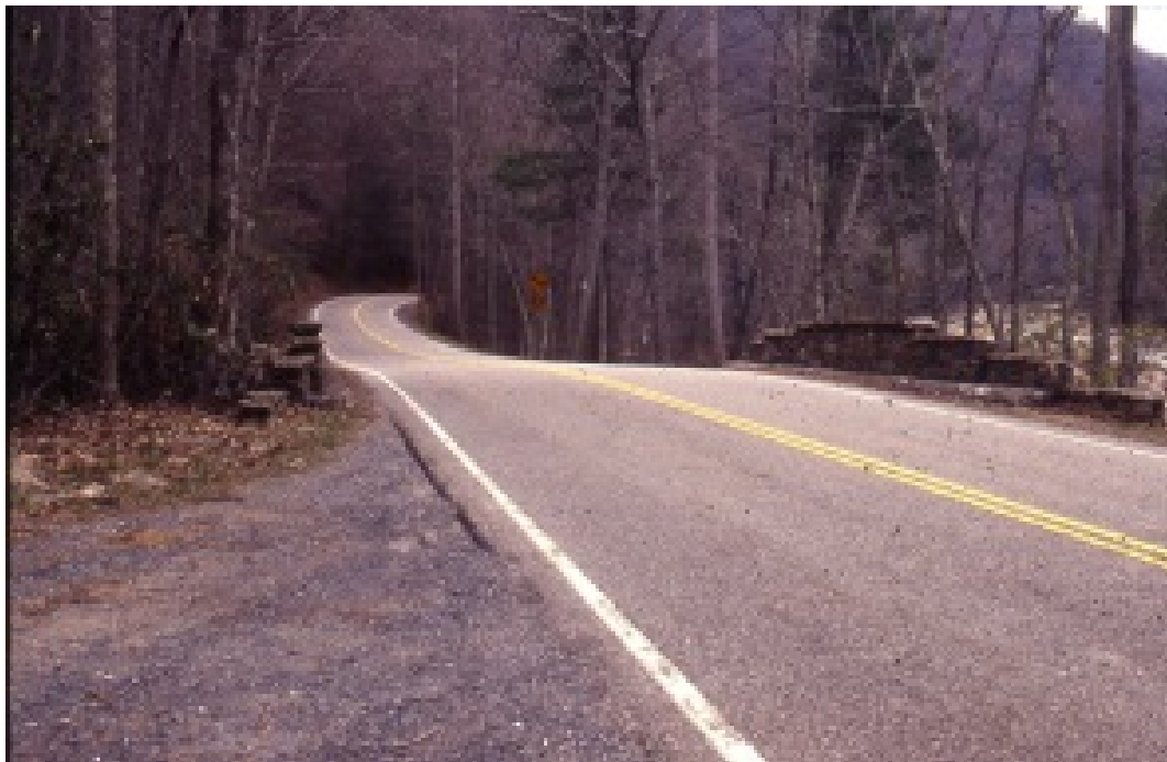
Figure A3. Goshen Pass: Route 39 at the Laurel Run Bridge
